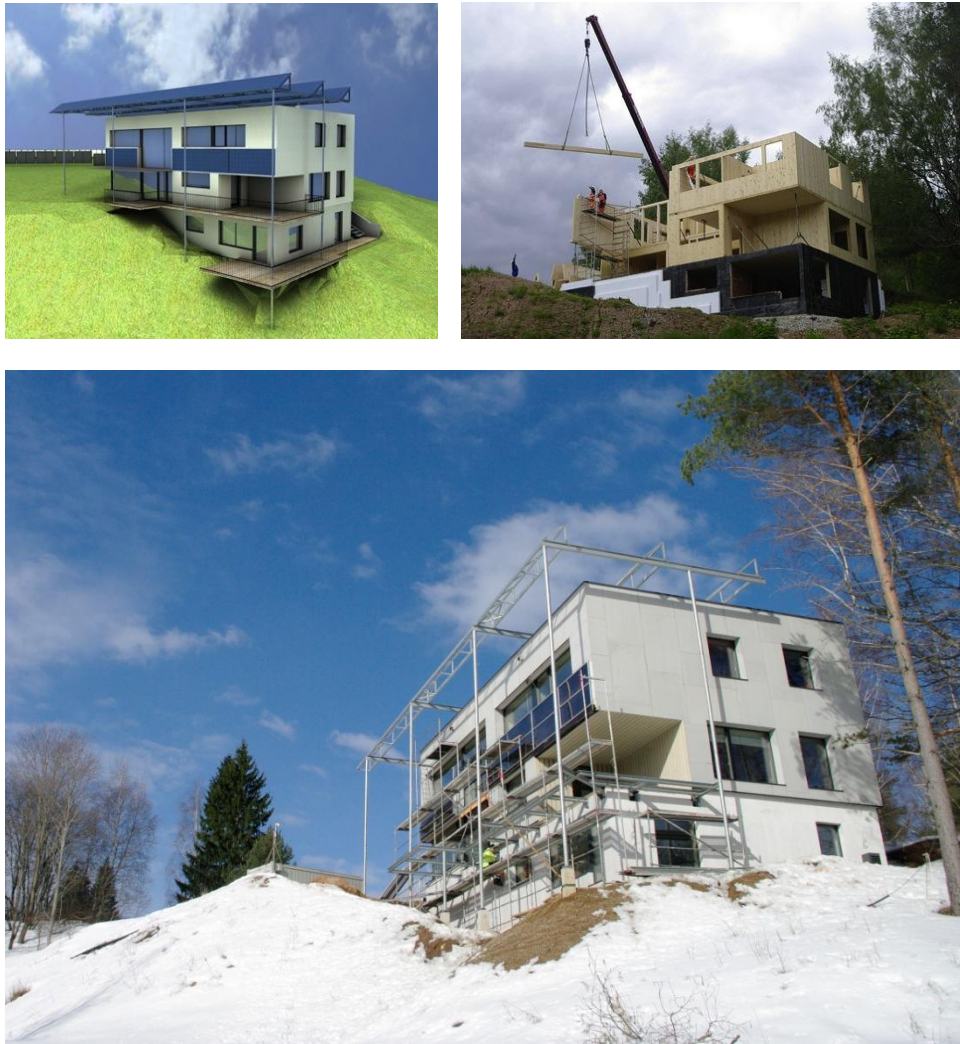
Figure 1 Rendered view and photos from building time.
